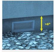
Embers accumulate against homes at the base of exterior walls and on other horizontal surfaces like decks that can ignite the home.
