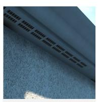
Because of their geometry, radiant heat can build up in an open eave and ignite exposed materials. Flames from nearby fuels such as a shed or vegetation can also ignite eaves.
